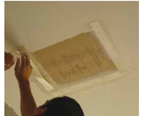
Installing Amina speakers
